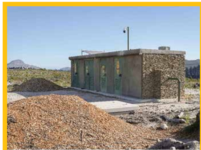
FIGURE 6: Completed pumphouse structure clad with natural stone to reduce visual impact
