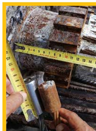
FIGURE 9: Comparing the existing couplers with the closest available match on the contemporary market
