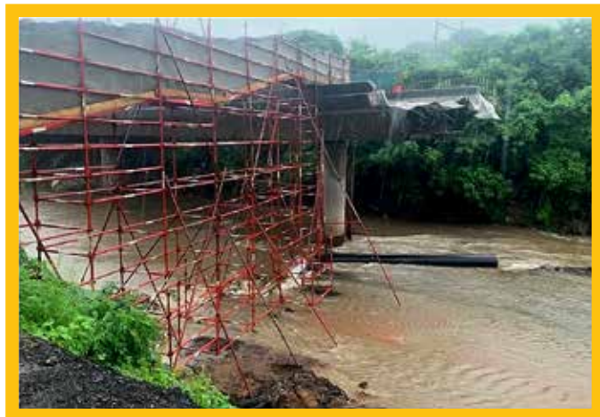
FIGURE 10: Temporary supports had to withstand repeated flooding
