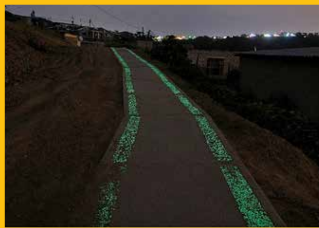
FIGURE 8: Illuminating sidewalks leading to the bridge
