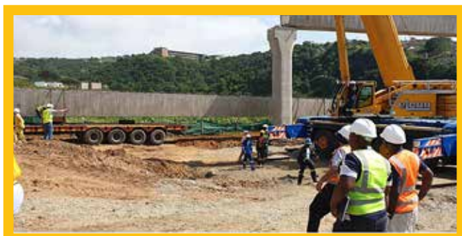
FIGURE 4: Installation of bridge decking
