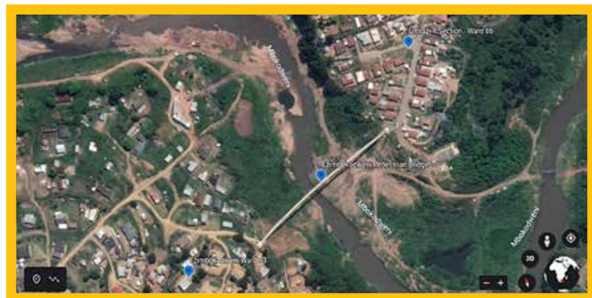
FIGURE 2: An aerial view of the site post-construction. The picture depicts the newly built bridge and the wards serviced
