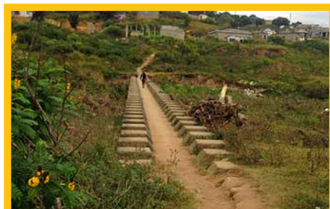
FIGURE 1b: The existing bridge prior to re-construction
