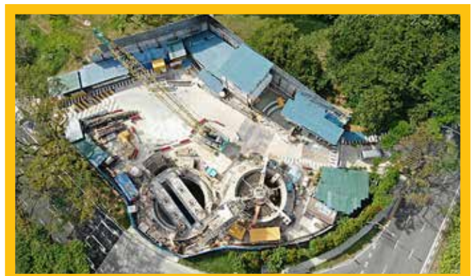
FIGURE 9: Aerial view of shaft sinking site
