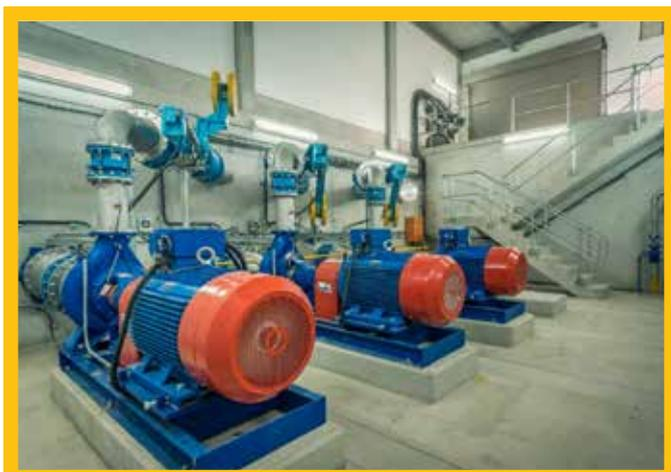
**FIGURE 11:** Lelifontein Pump-As-Turbines installed, with space for future unit in background
