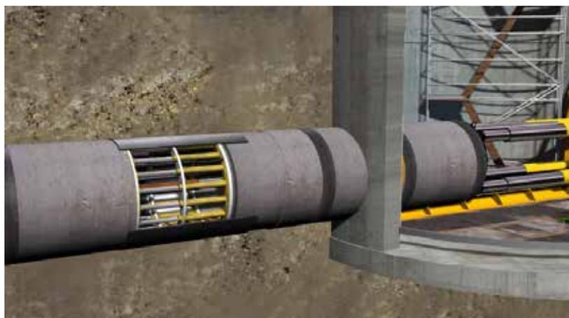
**FIGURE 6:** Interjacking station in operation.
