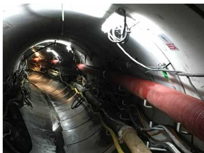
**FIGURE 14:** View in tunnel (ID 2 000) with curve radius of 110 m constructed in France
