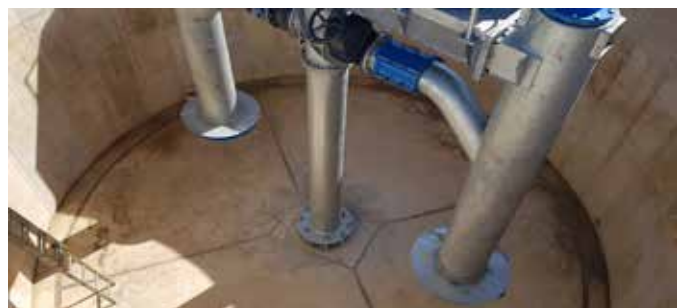
Picture 1.5: Kruisfontein Patented Transfer Mixer
