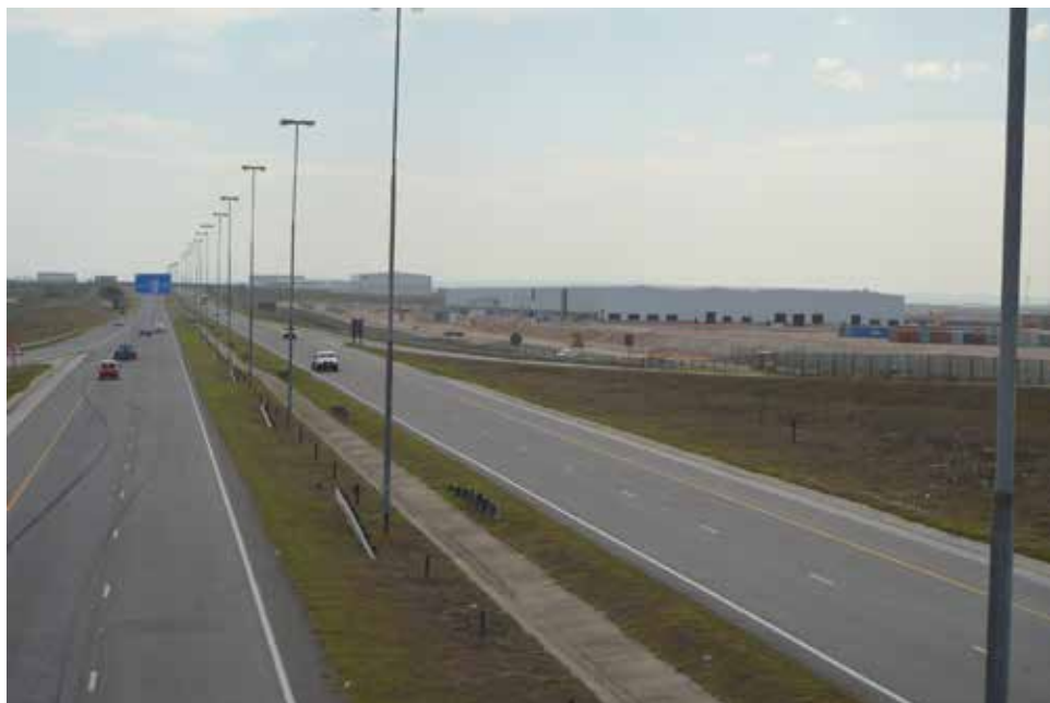
Figure 1: The Construction of the multi-billion rand factory by the Beijing Automobile International Corporation (right) at Coega SEZ is a good example of the pin-offs in public sector investment in enabling infrastructure. Pic by Ongama Mtimka.
