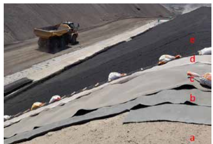
FIGURE 11. Installation of layers.
