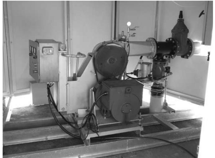
Figure 5: Cross flow turbine installation on top of old reservoir
