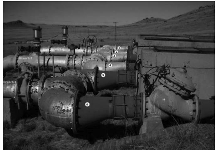
Figure 3: The six control valves on the 3 branches feeding into the Uitkijk Reservoir
