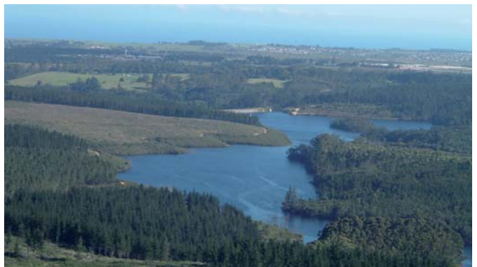
Figure 2 : Garden Route Dam – Full
