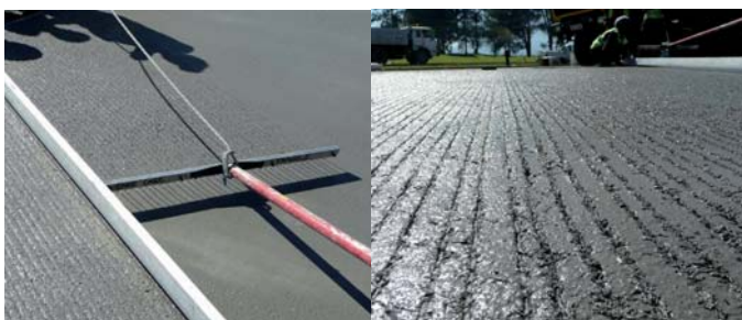
Figure 8: Texturing using tine grooving rake (left); final surface texture, 26 mm average spacing (right)
