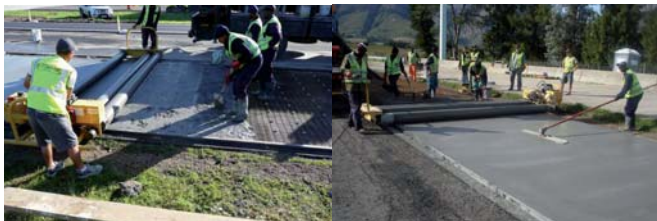
Figure 7: Triple-screed oscillating roller using square tubing side forms as rails
