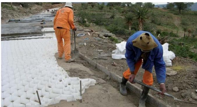
Figure 8 : Excavation of edge thickening
