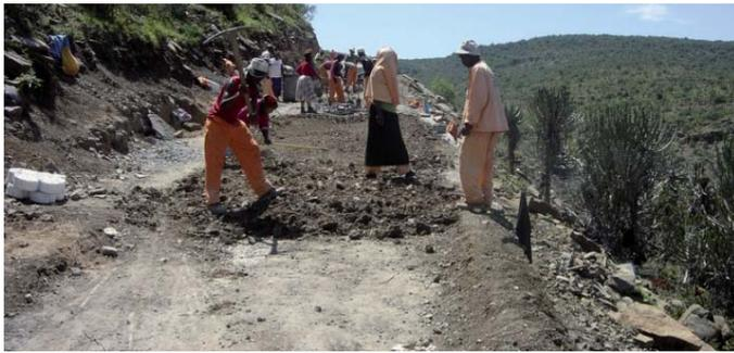
Figure 5 : Reworking insitu Material & Shaping road base
