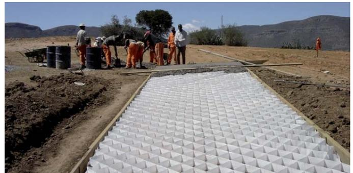
Figure 10 : Setting out geocells
