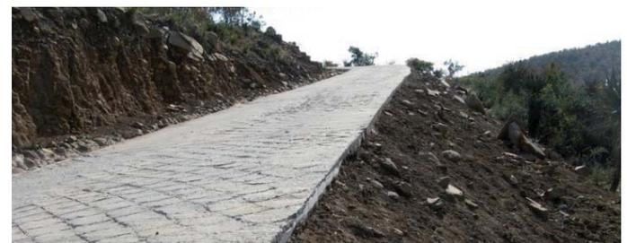
Figure 14: Exposed edge to geocells
