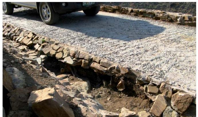
Figure 15: Erosion of stone-pitched drain
