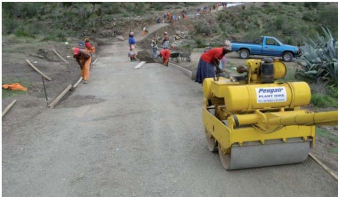
Figure 7 : Compaction of base layer
